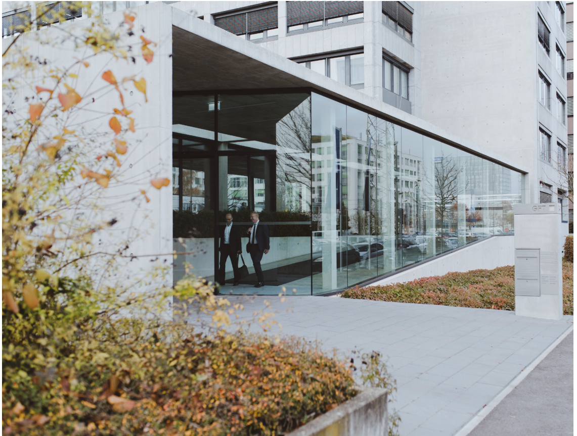
GFT Corporate Center in Stuttgart, Germany
